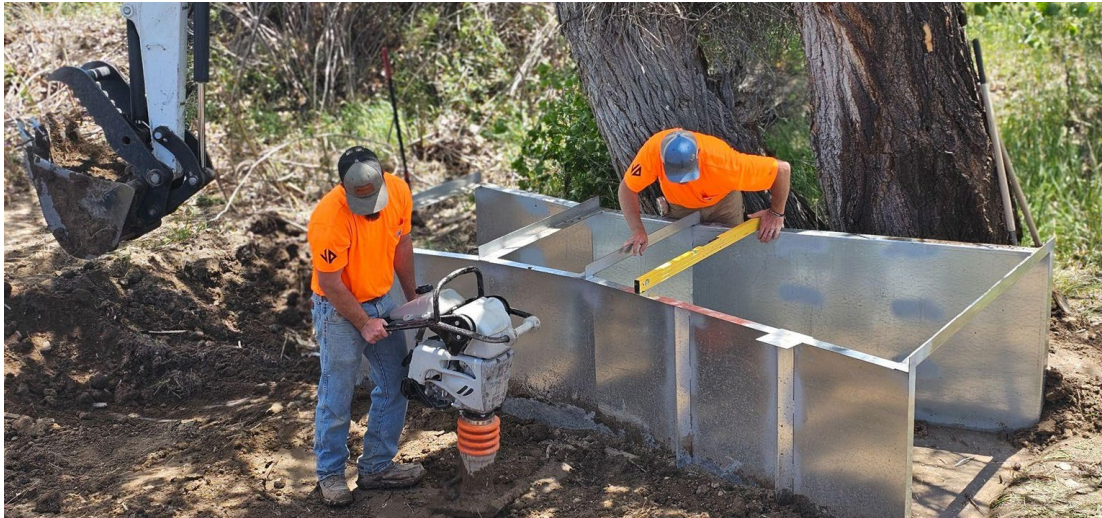
Flume Example for Return Flows - South Marsing Wash from the Carbon Canal
