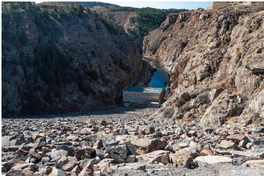
Blue Mesa Dam and Powerplant.
