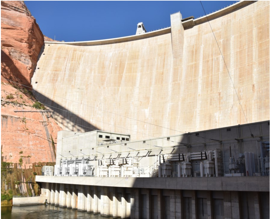
FIGURE 5. Transformer Deck at Glen Canyon Dam Powerplant
