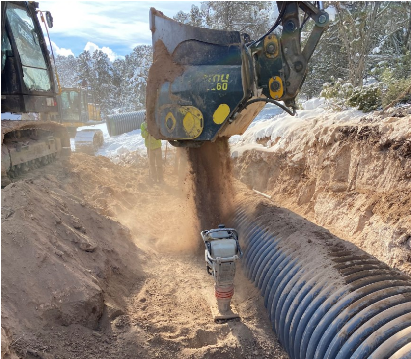
FIGURE 16. Backfilling Pipeline on Section Two of the Gould Canal Improvement Project B - in Crawford, Colorado
