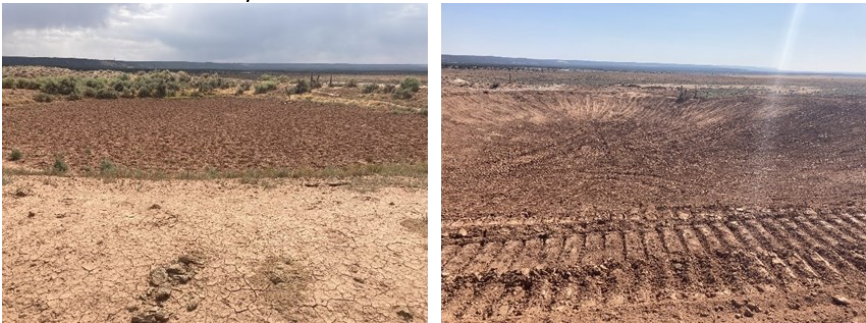
FIGURE 23. Farnsworth Reservoir in the Kanab Creek watershed before (left) and after (right) sediment removal.
