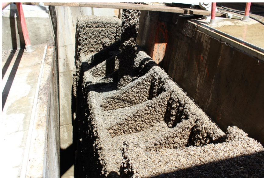
FIGURE 10. Quagga mussels accumulated on a fixed wheel gate pulled out of the water for maintenance at Glen Canyon Dam, Arizona. These nonnative species anchor themselves to nearly any surface near running water and reproduce rapidly. Mussel populations have covered boats, marina docks, motors, pipes and other water works in many Reclamation infrastructures, reducing the efficiency of these resources.
