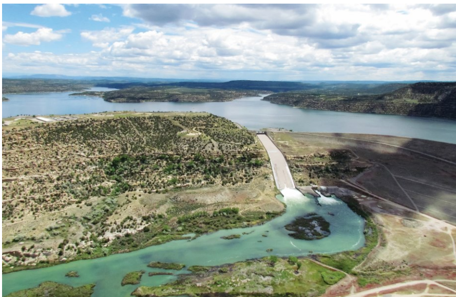
Figure 7. Water from Navajo Reservoir is released down the Navajo Dam spillway. The dam is located on the San Juan River, 34 miles east of Farmington, New Mexico. (Reclamation photo by S. Pernick)
