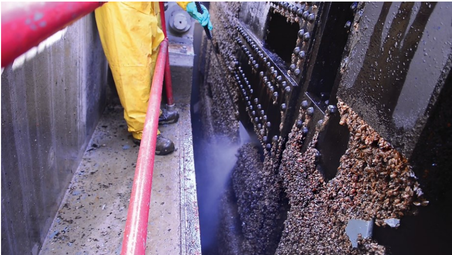
Figure 9. Reclamation maintainers power spray off Quagga and zebra mussels that cling to the sides of the metal surfaces on a penstock gate at Glen Canyon Dam, Arizona. These nonnative species anchor themselves to nearly any surface near running water and reproduce rapidly. Mussel populations have covered boats, marina docks, motors, pipes and other water works in many Reclamation infrastructures, reducing the efficiency of these resources. (Reclamation photo by Chris Watt.)
