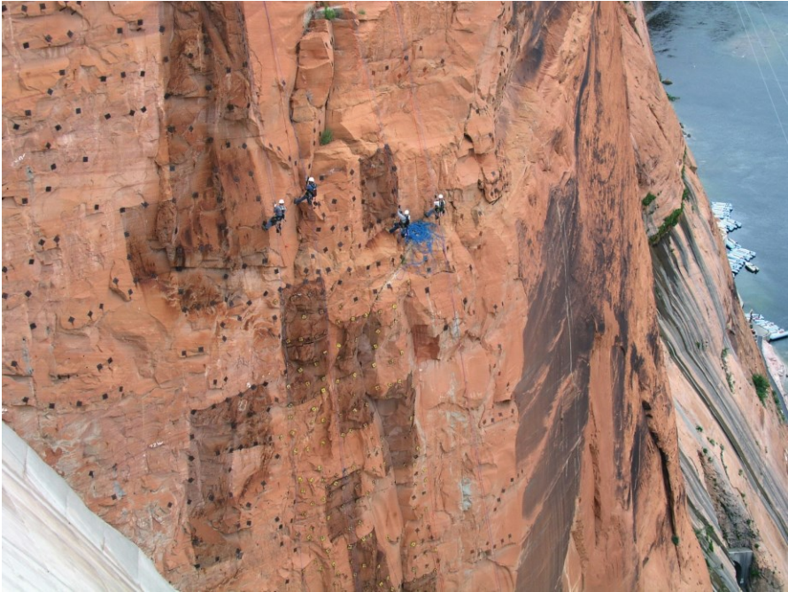
Figure 5. Reclamation professionals called high scalars, rappel down Glen Canyon walls, downstream of Glen Canyon Dam, Arizona. High scalars secure layers of Navajo sandstone by drilling and anchoring metal bolts up to 16-feet long, all while they are suspended hundreds of feet above the Colorado River. (Reclamation photo by Mark Neeley.)
